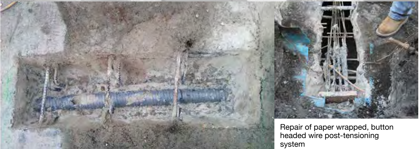
Inspection of grouted (bonded) post-tensioned tendon
